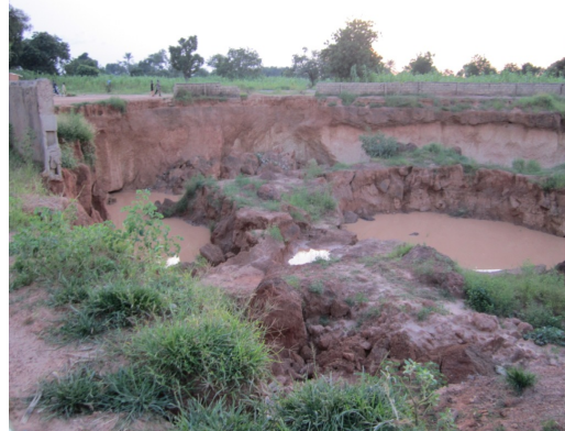
Plate 16: Erosion in Garandiya
