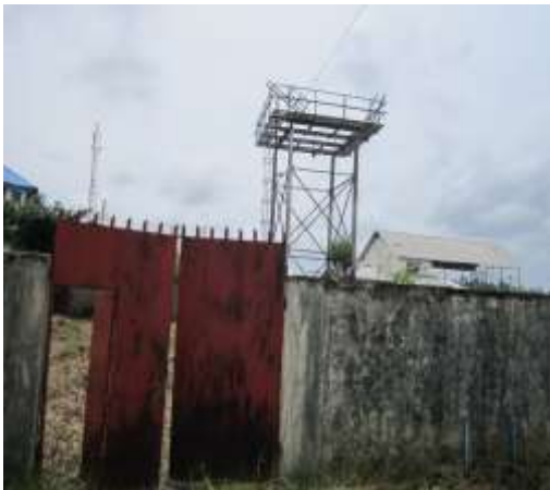
Plate 13: Soku community water supply Project (uncompleted)
