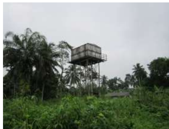
Plate 18: Uncompleted State Government water project
